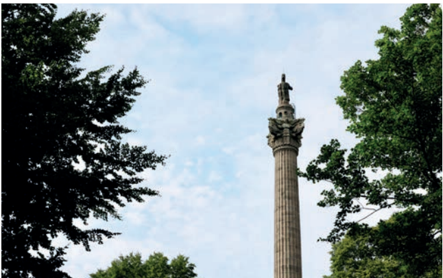
The $2.2 million restoration of Brock’s Monument is done.
