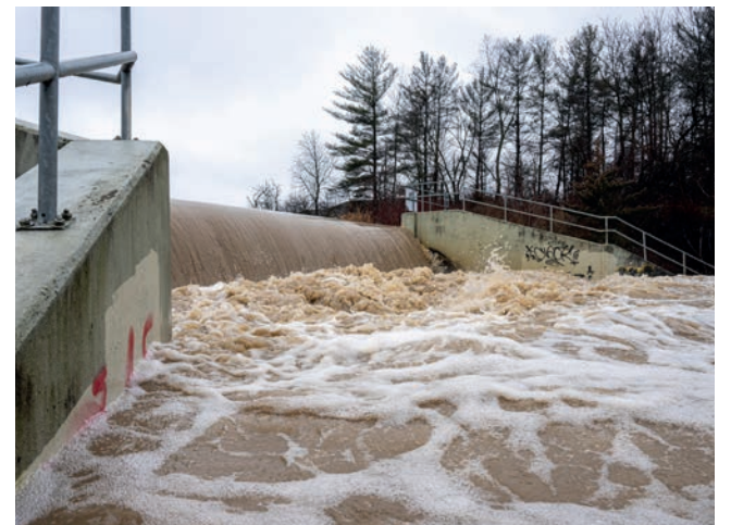
Flooding at the Virgil Dams along Four Mile Creek in 2024.
