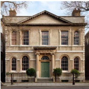
A balanced Georgian symmetrical façade.
