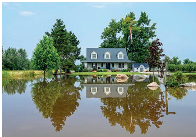
A flooded Niagara-on-the-Lake home after this summer's severe storms. Letter writer Christine Earl says trees, permeable surfaces and other “sponge city” measures could help reduce future flooding. FILE/DAVE VAN DE LAAR
