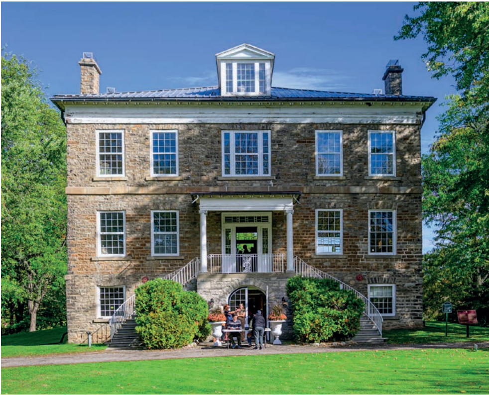
Since 2006, students have been receiving an education at the Willowbank school in how to preserve and restore buildings and other historic properties. The estate itself is a historic property dating back to the 1830s. FILE/DAVE VAN DE LAAR
