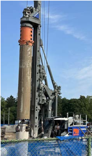
Caissons, a watertight steel tube that acts as a stable foundation for large structures, are being installed at the site of the future Parliament Oak hotel. BRIAN MARSHALL
