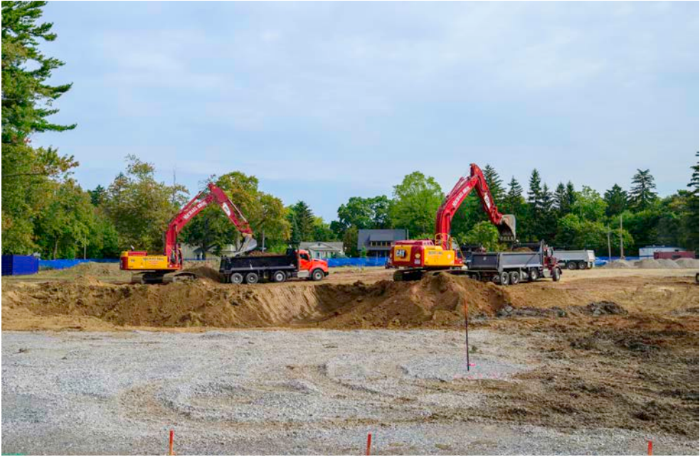
Trucks are illegally hauling dirt from the Parliament Oak site, despite a stop-work order from the Town of Niagara-on-the-Lake on Tuesday. DAVE VAN DE LAAR
