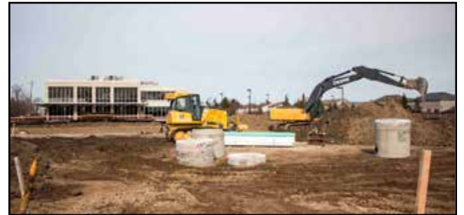
Construction has started at 1561 Niagara Stone Rd. in Virgil. (Richard Harley)
