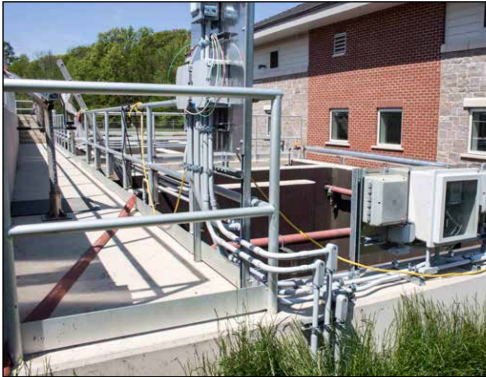
The wastewater treatment plant on Lakeshore won't be open until November. (Supplied)
