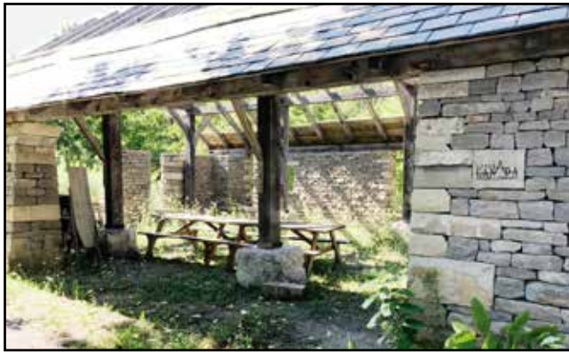
The Drystone Wall building. (Lauren O'Malley)
