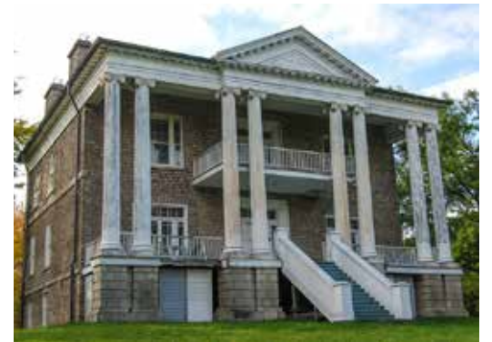
Portland brick damage. (Supplied photo)
