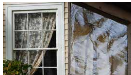
A six-over-six window with early-cylinder glass pane. (Supplied photo)
