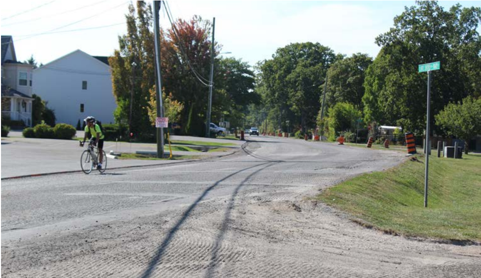
Construction will continue on Lakeshore Road and Mary Street until Sept. 30. DAN SMEENK
