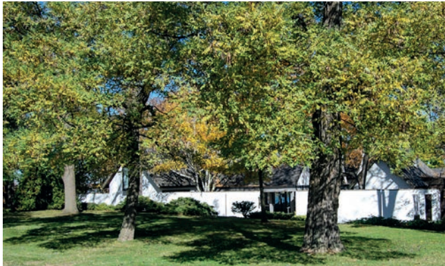
The Chapman House, a mid-century modern home on the Niagara Parkway, has been relegated to “the dustbin of history” by the town's approval of its demolition, writes Brian Marshall. And it's hurting NOTL's heritage. FILE
