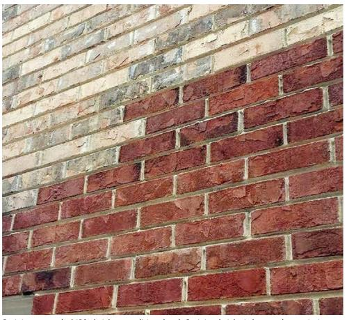
Staining a mottled '80s brick to traditional red. Staining bricks is better than painting, allowing the brick to retain its necessary porous quality, Brian Marshall writes. SUPPLIED
