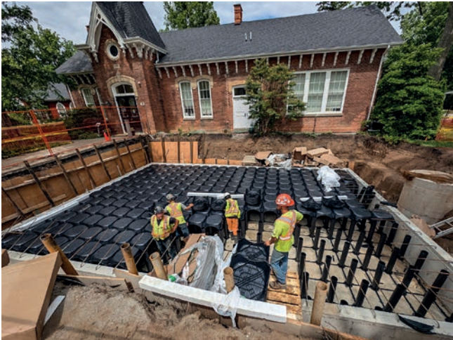
As part of the Niagara-on-the-Lake Museum’s expansion, underway right now, it’s adding a detention tank to temporarily store stormwater when it rains — Brian Marshall says it’s the responsible choice. BRIAN MARSHALL
