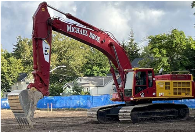
An excavator is ready to dig a 23-foot hole at Parliament Oak to accommodate underground parking. GARTH TURNER
