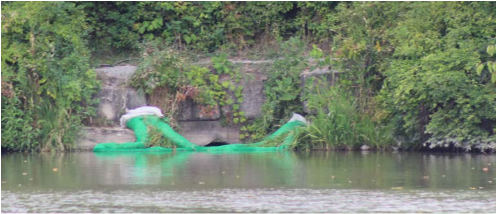
Absorbent pads were used to remove oil that entered the reservoir. DAN SMEENK
