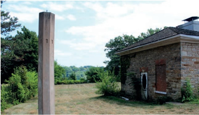
The stone schoolhouse (and its chimney) on 14785 Niagara River Pkwy., built in the 1830s. FILE/DAN SMEENK
