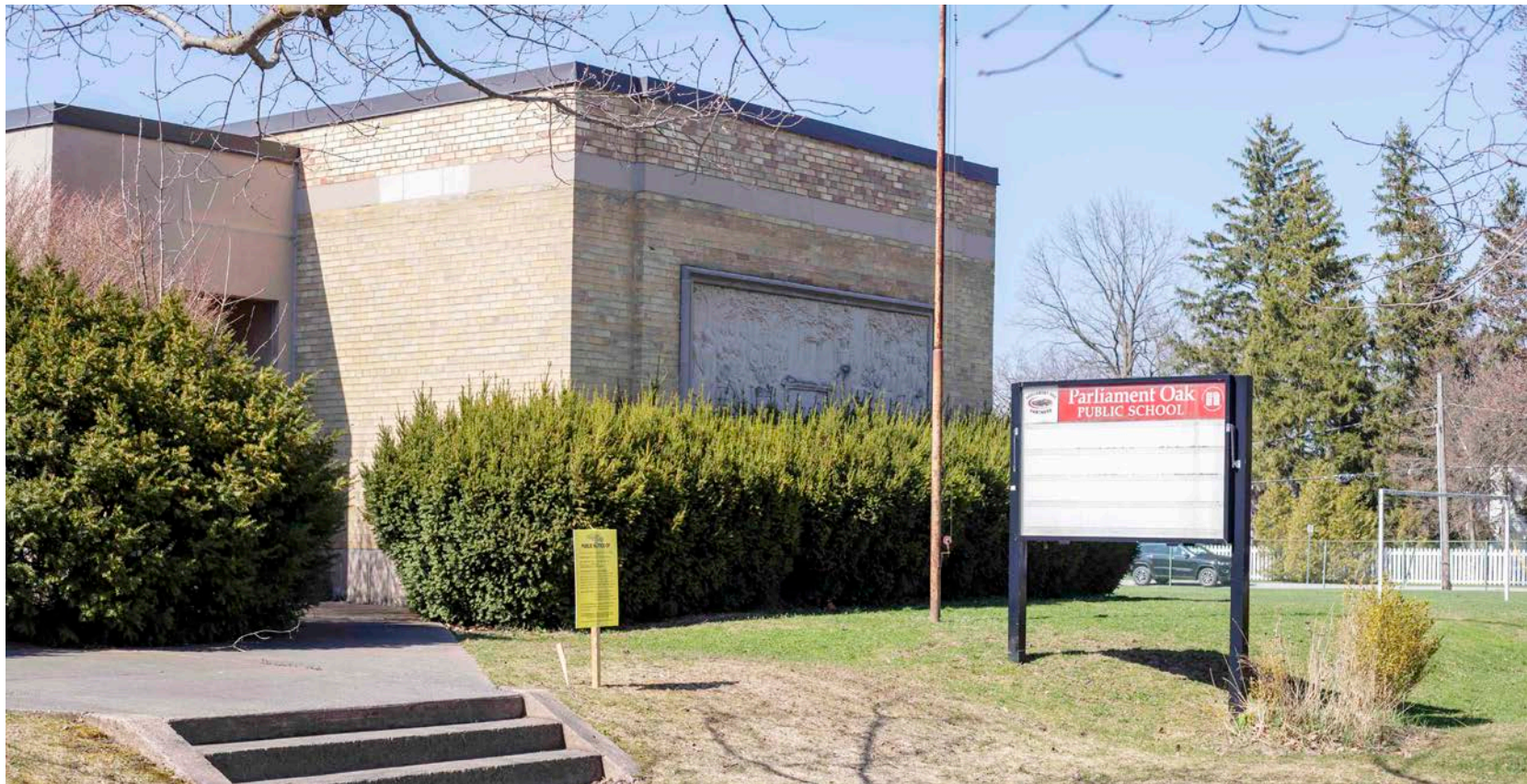
Two Sisters Resorts Corp. has plans to demolish the old Parliament Oak school with intentions to preserve some of its heritage features EVAN LOREE
