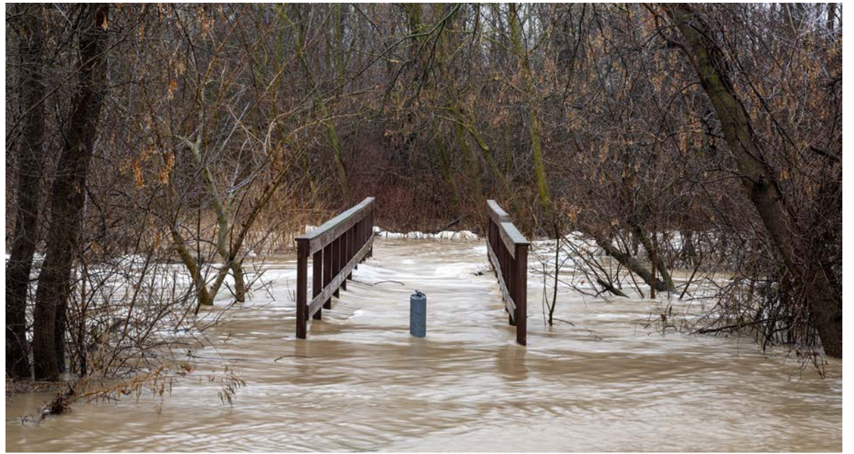
Photographer Dave Van de Laar captured this image of flooding at the dam on Line 2 Road on Jan. 26.
