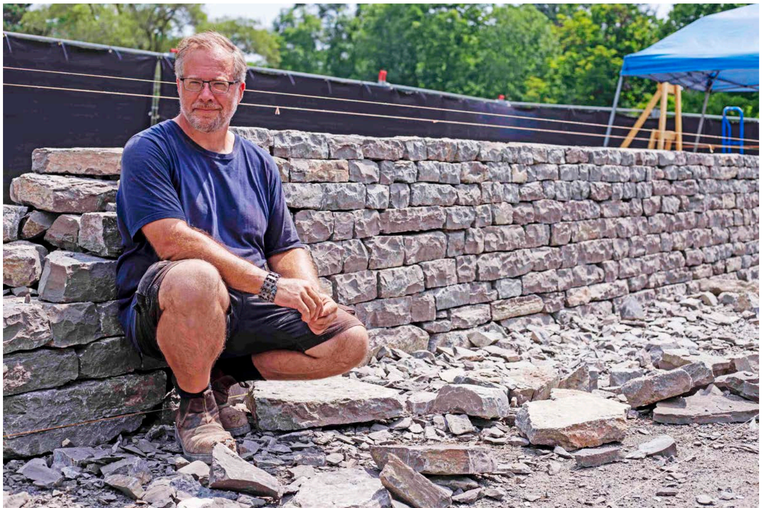
Menno Braam, a dry stone mason, is building the town's new drystone wall gateway sign. Story on Page 3. EVAN LOREE
