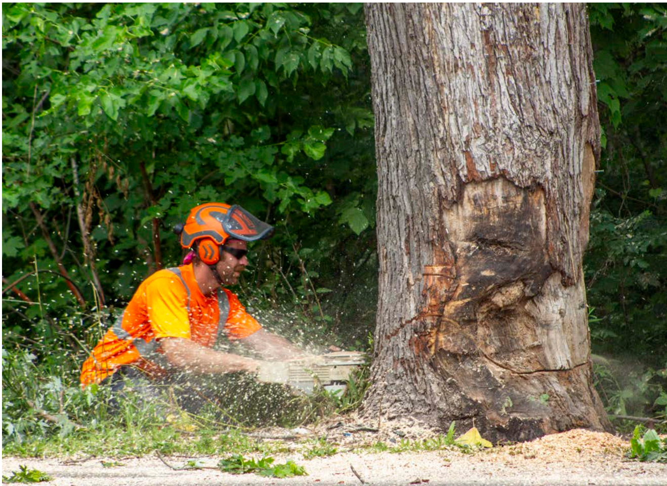
Workers from Safe Tree Ltd. took down the Lakeshore Road mature tree on Wednesday morning, starting with individual branches before removing the base of the tree. A crowd gathered to watch the cutting. JULIA SACCO
