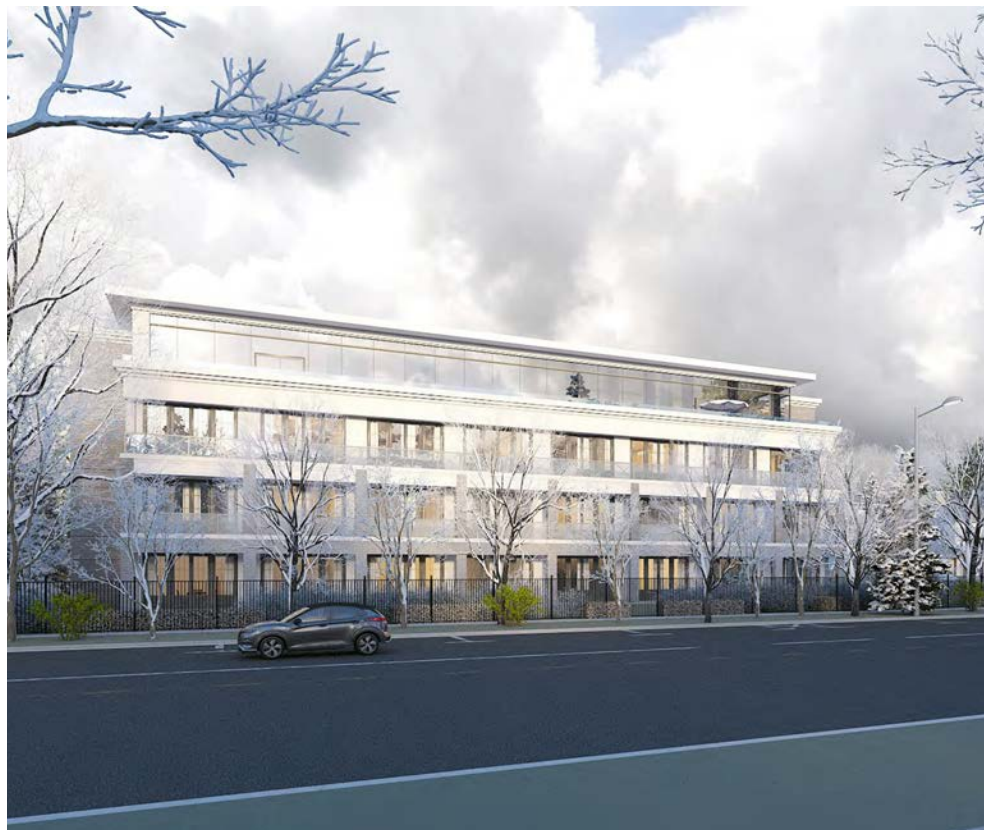
The four-storey hotel proposed by developer Rainer Hummel for Queen Street — if built according to modernist drawings such as this submitted by the applicant — will "fundamentally" alter the streetscape in Old Town, writes Brian Marshall.
