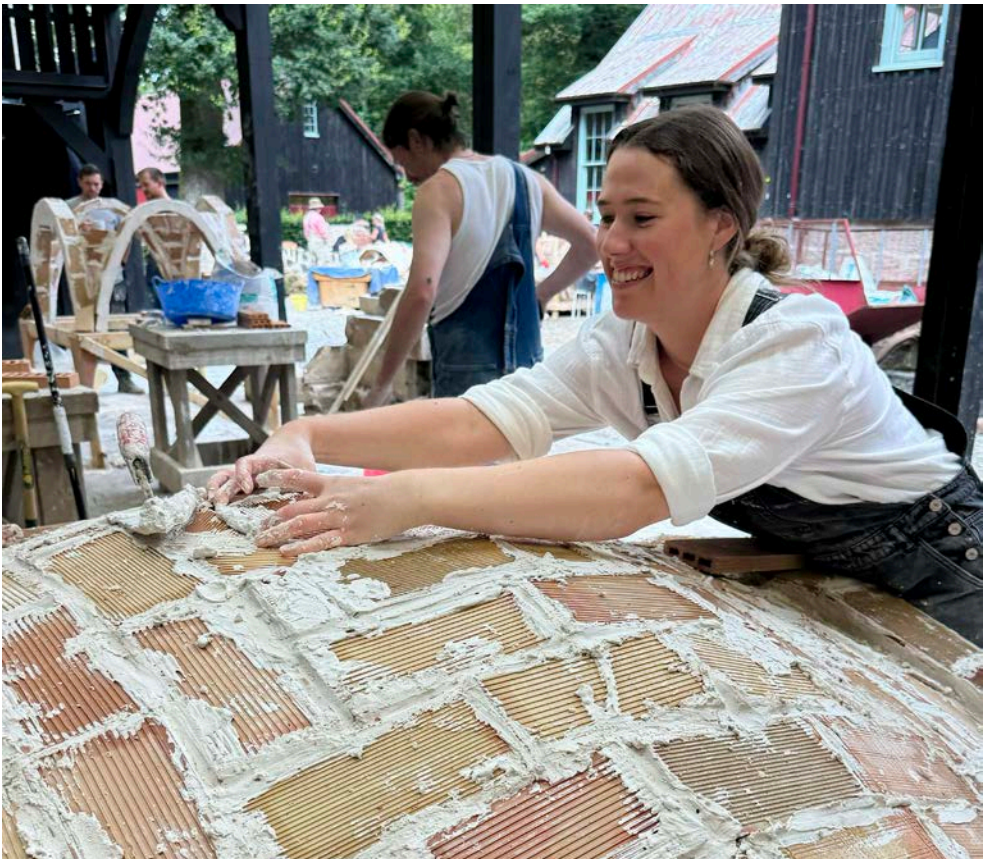
Julia Hodgson at Dumfries House creates a sail vault using thin clay tiles. Tile vaults derive their strength from their geometry rather than the material used. SUPPLIED
