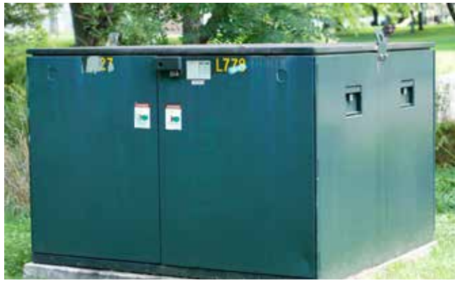
A hydro box near Memorial Park. BRITTANY CARTER
