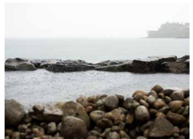
A new rock groyne to protect the dock area can't be installed until after fish spawning season is over in July. BRITTANY CARTER/FILE PHOTO
