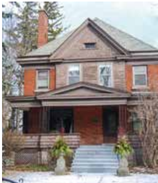
Edwardian missing its original columns but leaded glass still in place. SUPPLIED
