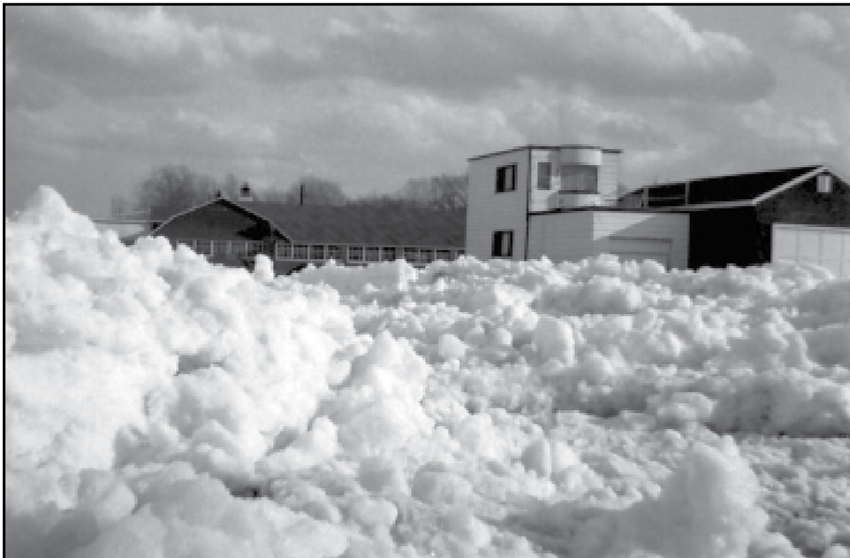
At the end of March 1955 the Niagara river was completely jammed with ice 50-feet thick above the waterline. Two houses, ten cottages and numerous docks and boat houses were completely destroyed. The picture shows the ice in the entrance to the Niagara marina with two boat houses and Shepherd boat works in the background.
