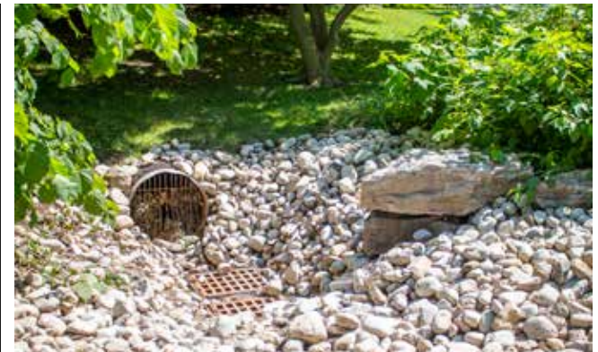
A bioswale at Simcoe Park is helping to filter out E. coli bacteria from storm drains in town. SUPPLIED
