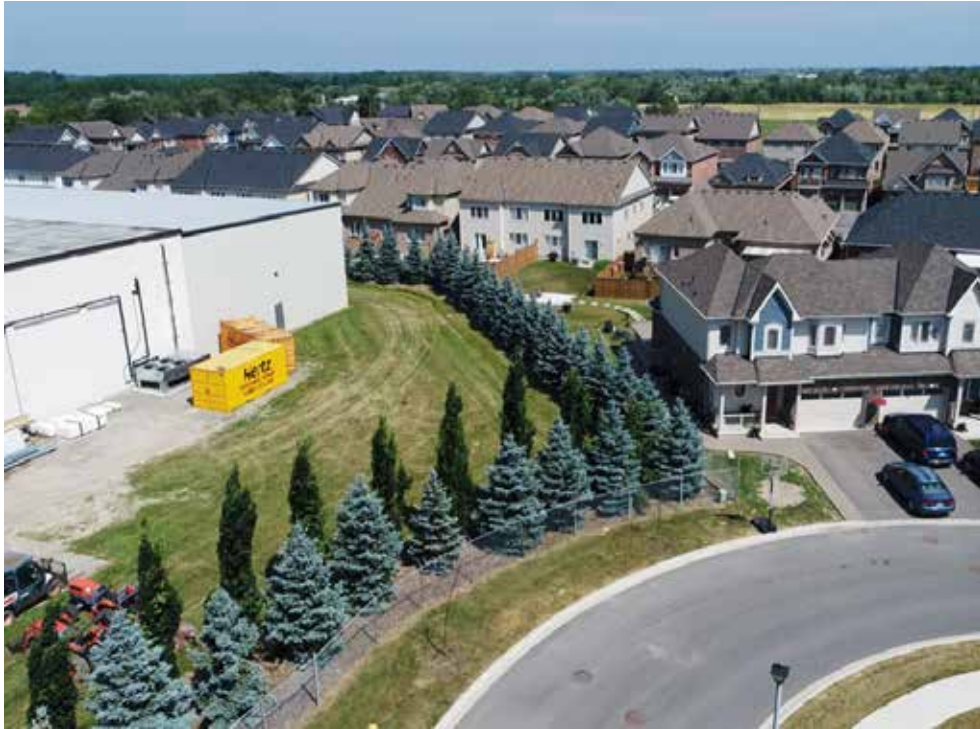
An aerial view of St. David’s Cold Storage, where nearby residents say noise from an air-conditioning unit is causing a bother. RENE BERTSCHI/SPECIAL TO THE LAKE REPORT
