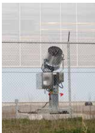
An outdoor turbine used by Canopy Growth to mitigate cannabis odour. DARIYA BAIGUZHIEVA
