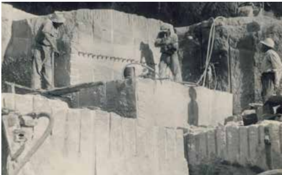
Men at work in the Queenston Quarries. KATHY THOMAS VIA VITACOLLECTIONS.CA
