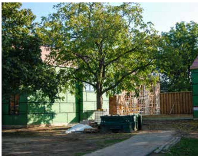
Another example of why NOTL needs design oversight. SUPPLIED/BRIAN MARSHALL
