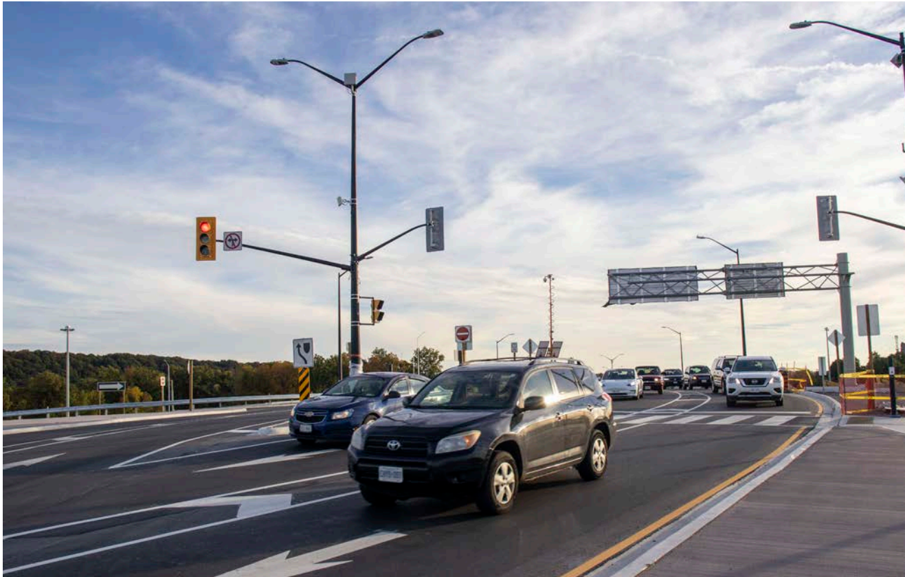
Cars drive through the new diverging diamond interchange in Glendale. Currently the off-ramp from Toronto is closed, as is the Toronto-bound on-ramp. SOMER SLOBODIAN
