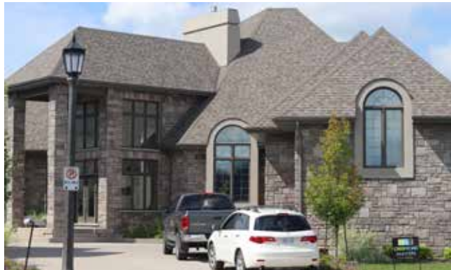
The exterior of a house on 31 Kenmir Avenue, which was targeted in drive-by shooting last Sunday, was damaged. DARIYA BAIGUZHIEVA
