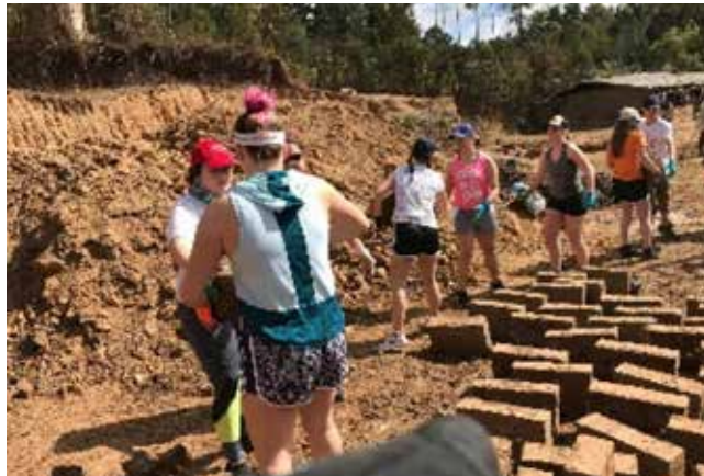
Volunteers move adobe blocks for building houses. SUPPLIED PHOTO
