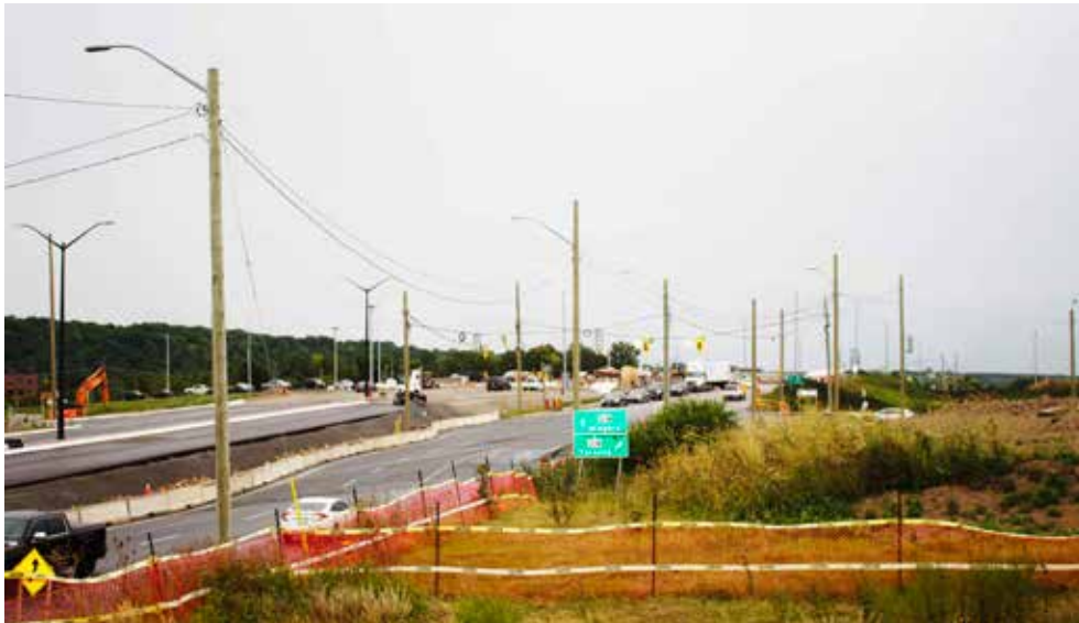
The new diverging diamond interchange in Glendale is confusing. FILE/EVAN LOREE
