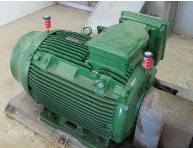
Application Electric motor Lubricator perma FLEX125 Installation kit Direct mount
