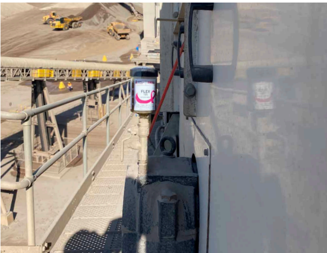
Application Conveyor pulley bearing and seal Lubricator perma FLEX125 Installation kit Direct mount
