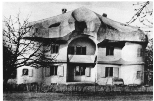
Fig. 5. Rudolf Steiner, Haus Duldeck, Dornach, 1915–1916. View from northeast (© Verlag am Goetheanum, Dornach).
