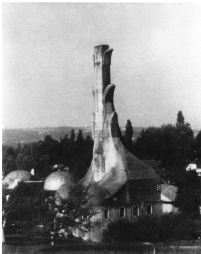
Fig. 6. Boiler House. View from south (author).
