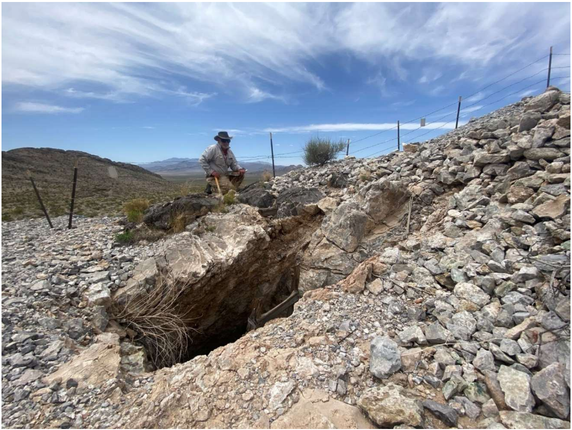
Photo 5: Top of inclined shaft, Desert Valley prospect. Note submeter-scale offsets of the black limestone hanging wall against the buff dolomite footwall.
