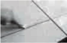
Before grouting, remove excess adhesive & debris from the joints.
