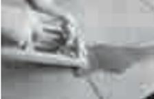
Fill the tile joints with the SpectraLOCK® Pro Premium Grout using a rubber float.
