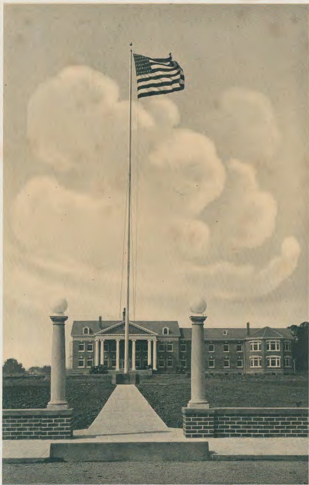
ADMINISTRATION BUILDING FROM TUALATIN VALLEY HIGHWAY, 470 FEET DISTANT.
