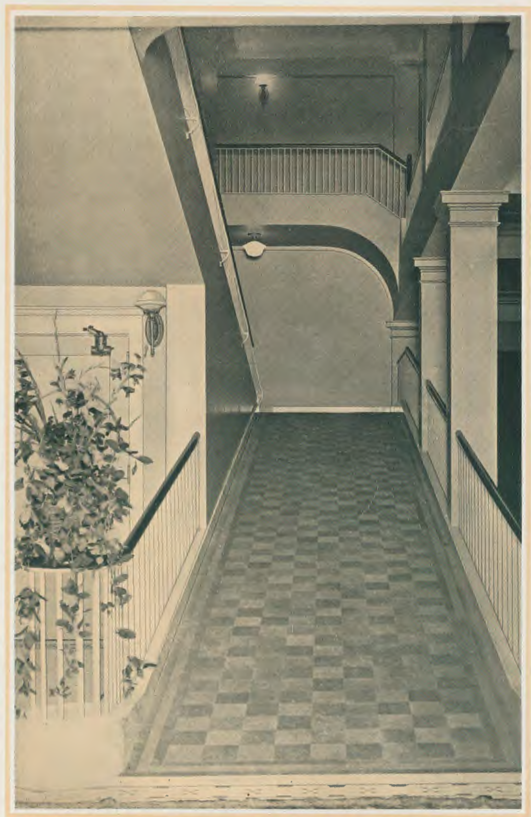
FROM THE LOBBY A REINFORCED CONCRETE INCLINE WITH ÇORK SURFACE LEADS TO THE SECOND FLOOR.
