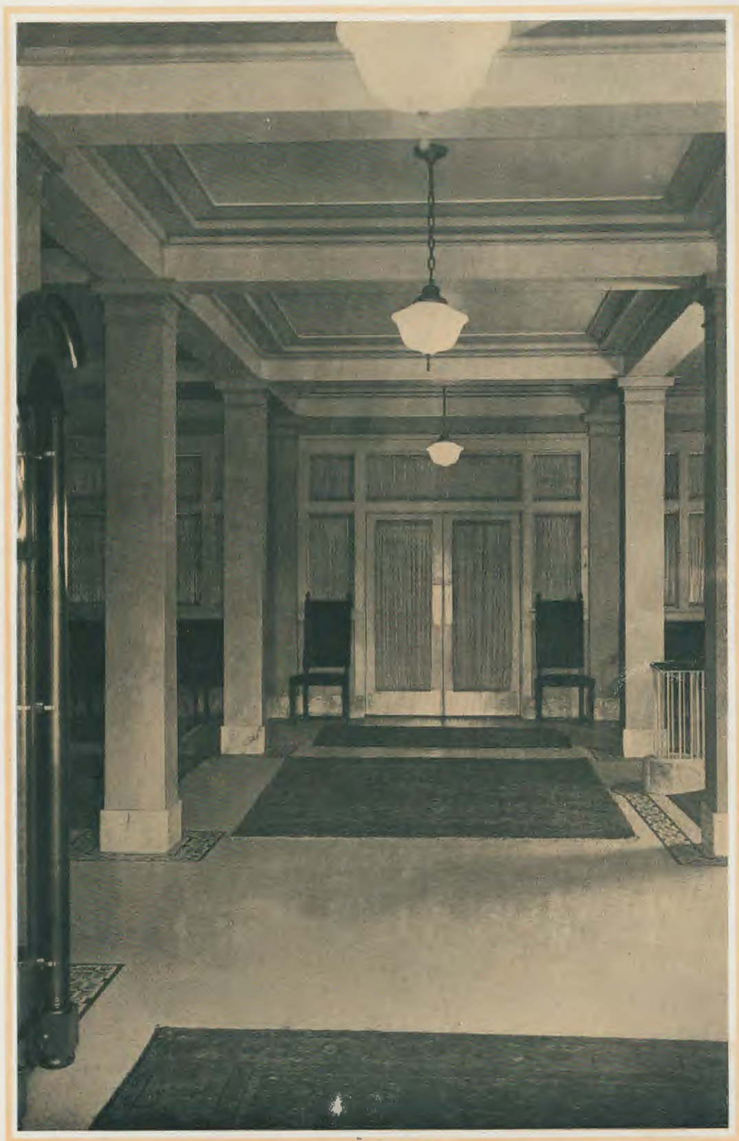
LOBBY, FROM MAIN ENTRANCE, LOOKING TOWARD DINING ROOM.
