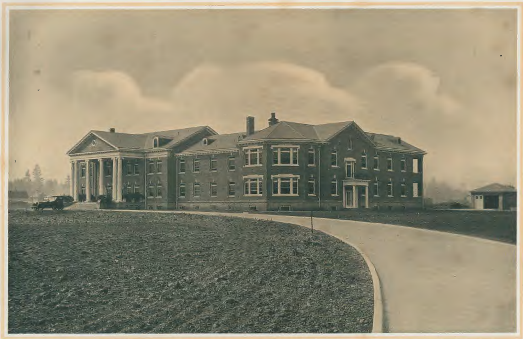
ADMINISTRATION BUILDING AND GARAGE FROM PRIVATE DRIVEWAY. THE BUILDING IS OF REINFORCED CONCRETE, BRICK AND TILE CONSTRUCTION.
