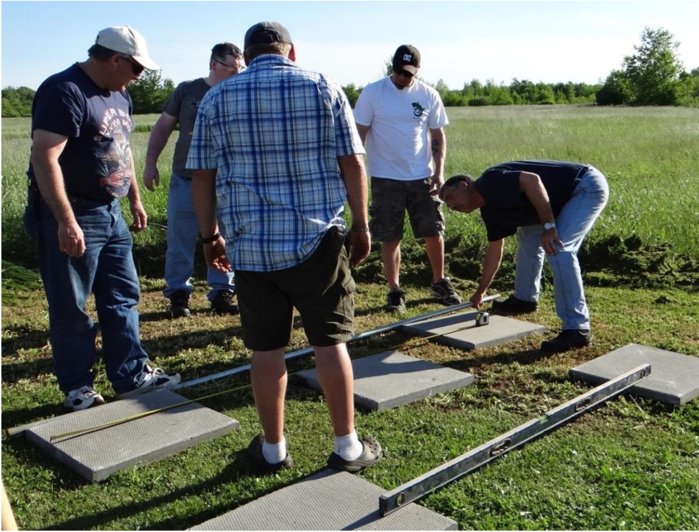
Figure 11 Leveling the blocks
