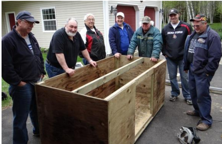
Figure 3 Lower compartment framed up
