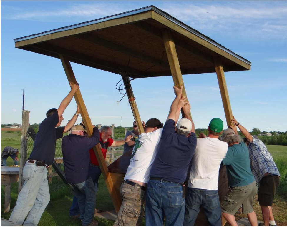
Figure 15 Raising the system
