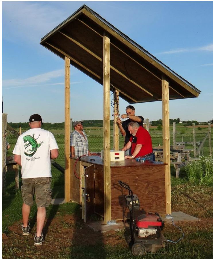
Figure 16 Bolt down and final wiring
