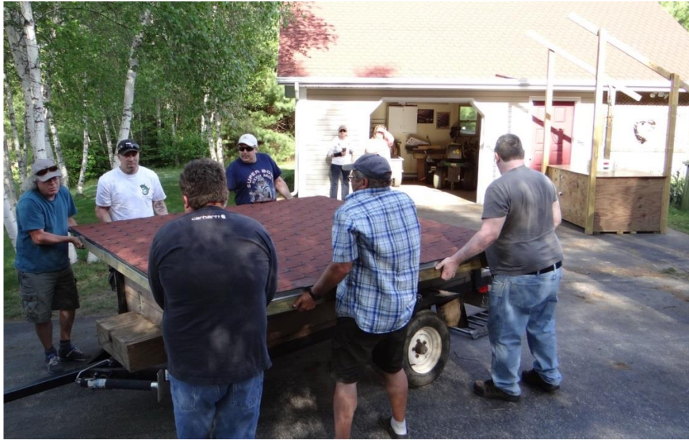
Figure 9 Loading the roof
