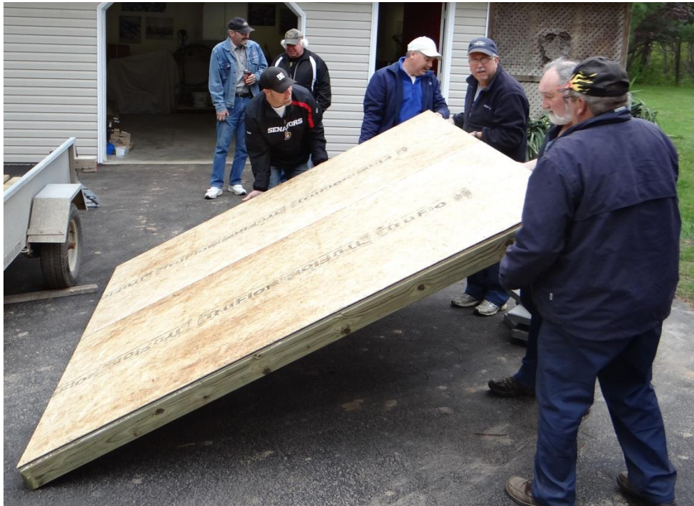
Figure 1 Roof framed up
