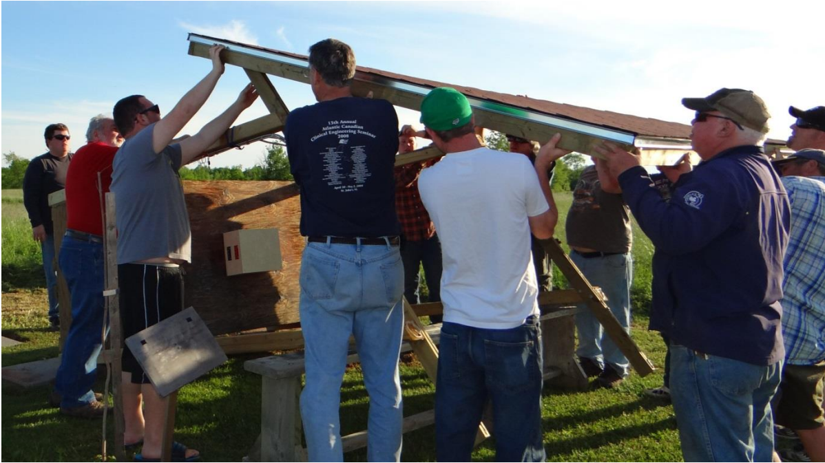
Figure 13 Installing the roof – industrial glue and very long screws
