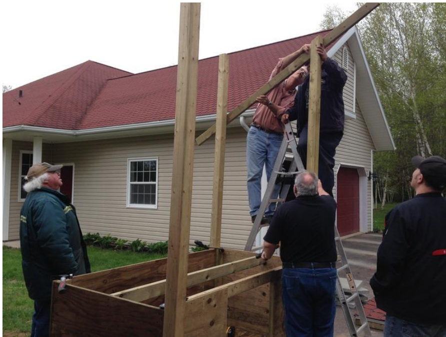
Figure 4 Roof supports going up and getting 30 degrees dialed in
