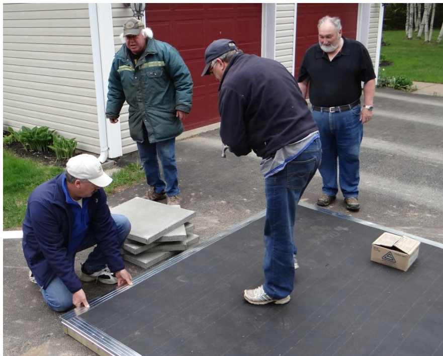
Figure 2 Tar paper and drip edging installed
