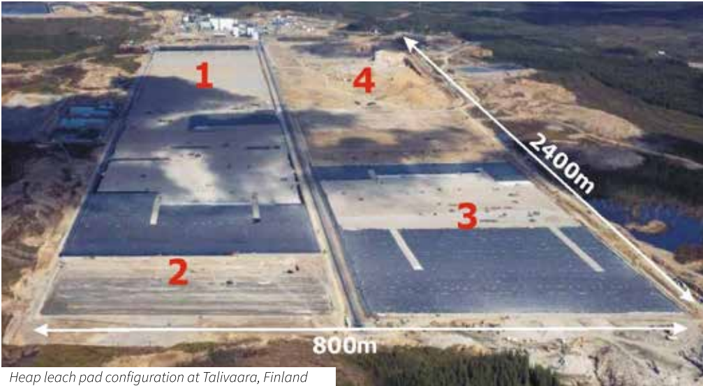
Heap leach pad configuration at Talivaara, Finland
