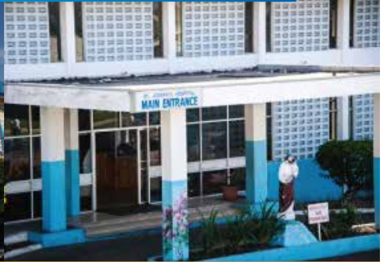
Princess Margaret Hospital, Montego Bay
