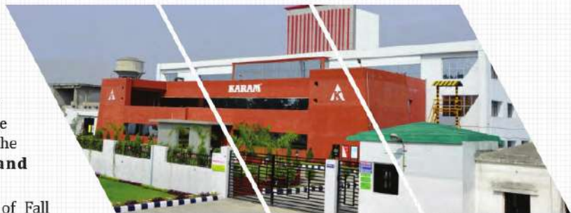
Unit-III Producing Helmets, Shoes, Fall Protection, Eye Protection, Ear Protection & Welding Protection - Sitarganj (Uttarakhand)
