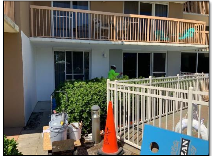
FIGURE 2 - Overall view of coating application in progress at ground floor mockup.
