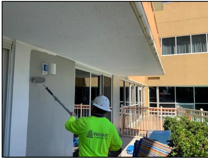
FIGURE 3 - Overall view of mockup location.
