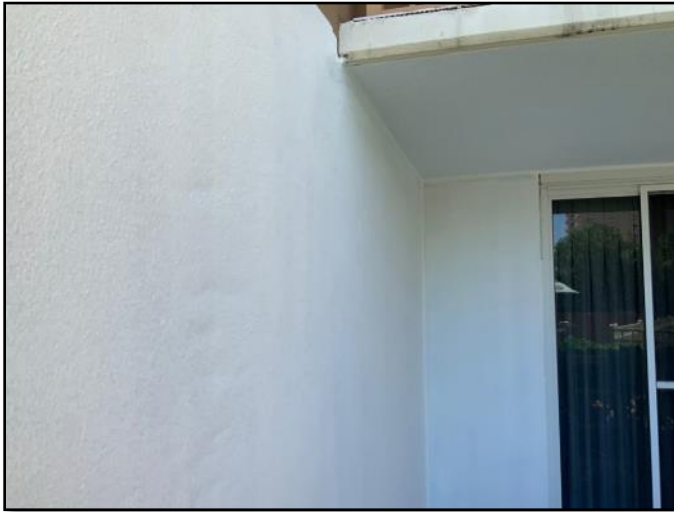
FIGURE 1 - Overall view of primer application at ground floor mockup.
