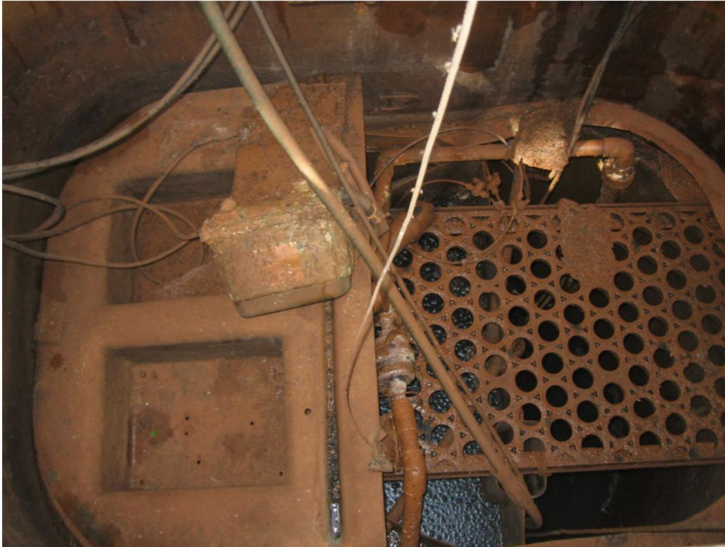
Pic 7 – inside ATU (left one in pic 3); green hose into ATU chamber; missing electrical components at left
