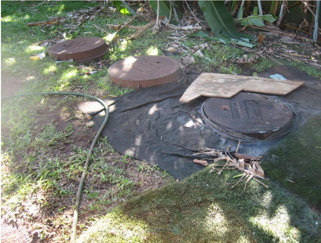
Pic 1 – Grease traps; grease trap overflow from first cover at right
