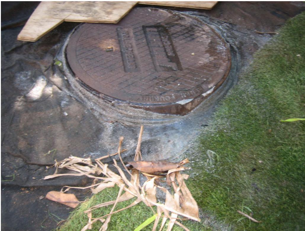
Pic 2 – close-up of active flow from grease trap
