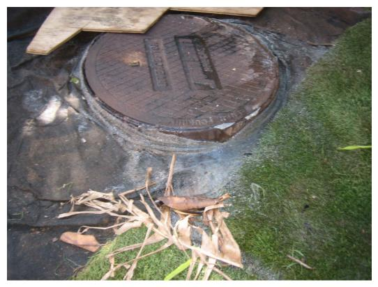
Pic 2 – close-up of active flow from grease trap
