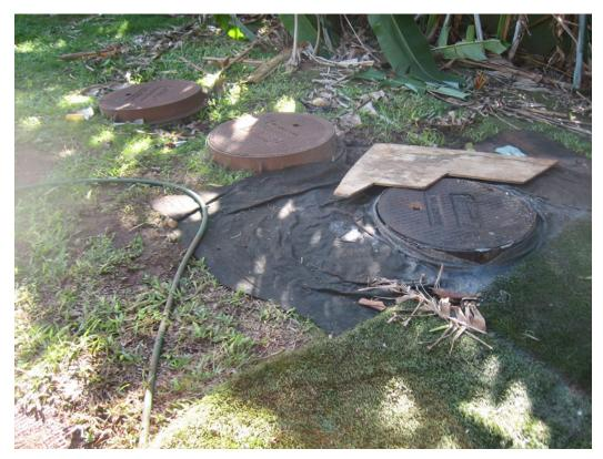
Pic 1 – Grease traps; grease trap overflow from first cover at right
