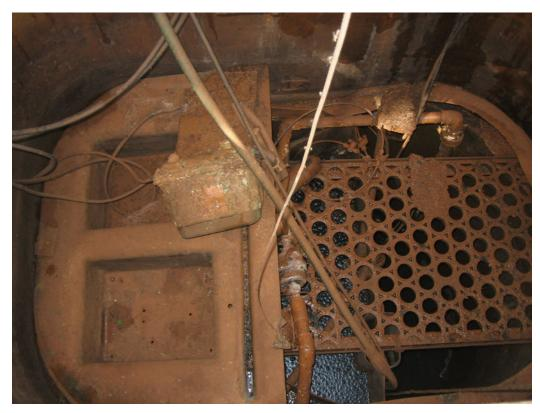
Pic 7 – inside ATU (left one in pic 3); green hose into ATU chamber; missing electrical components at left
