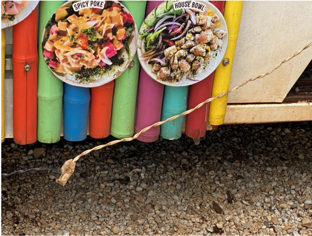
Electrical Code Photo 41
