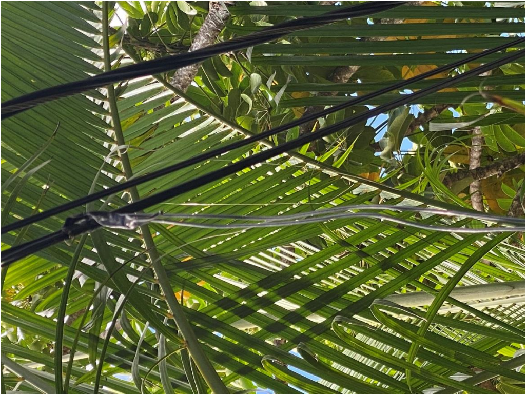
Electrical Code Photo 24
