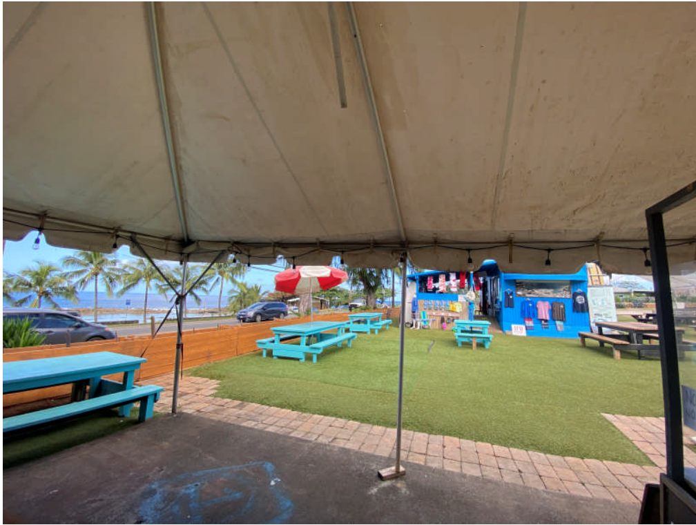
Electrical Code Photo 13
