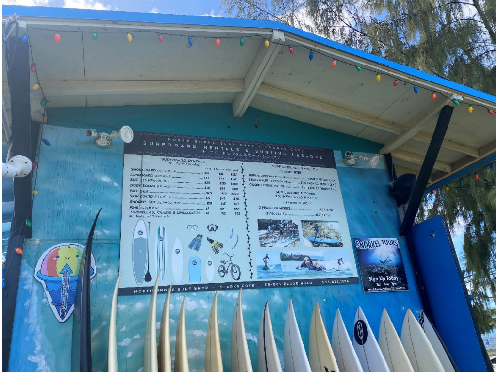
Electrical Code Photo 9
