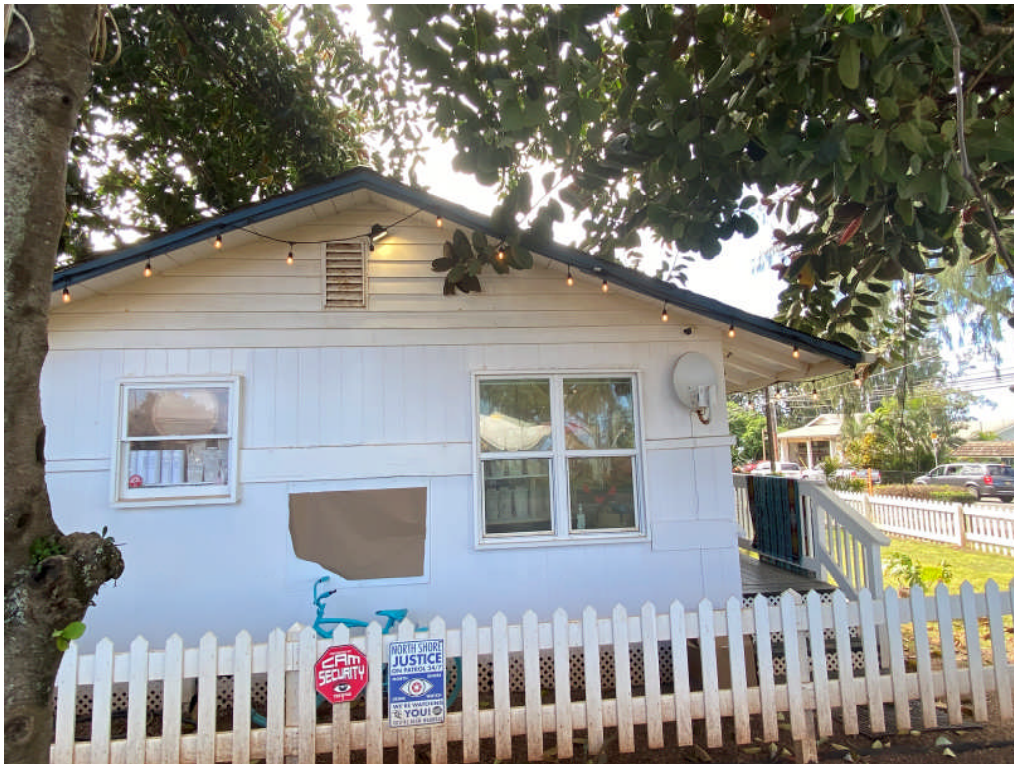
Electrical Code Photo 20
