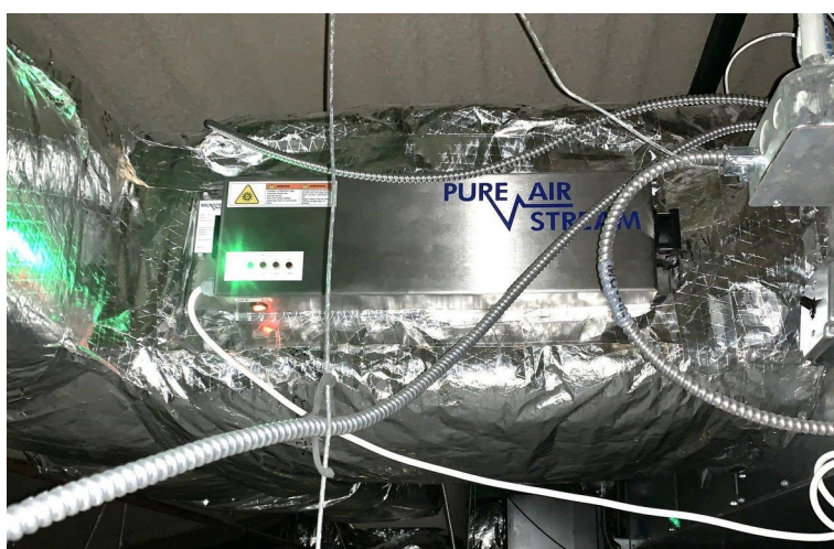
A PureAir Stream unit installed within an existing HVAC duct run.
