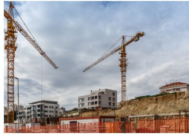
Construction Job Site
