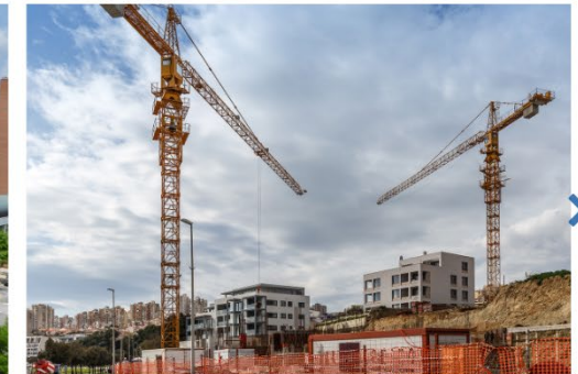
Construction Job Site
