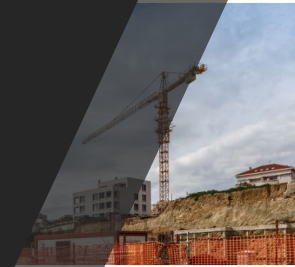
Construction Job Site
