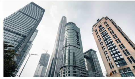
Office Building Job Site
