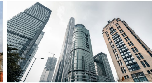
Office Building Job Site
