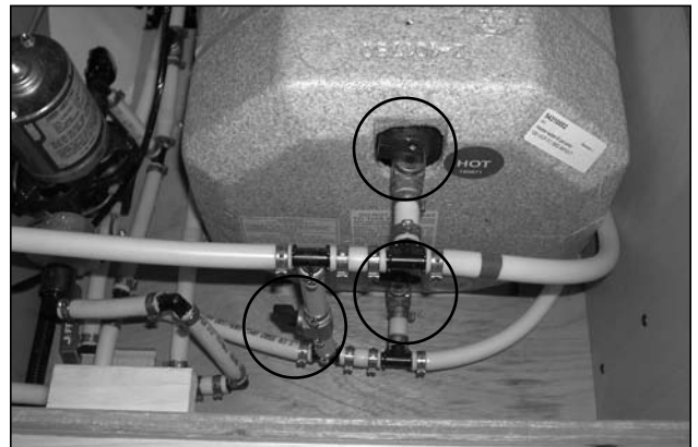
Picture G-P15: Winter mode valve positions.
